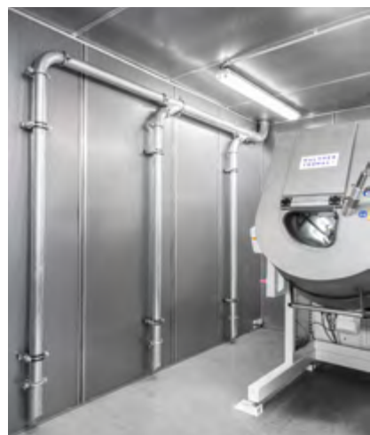
Optional sound enclosing cabin with air extraction system
