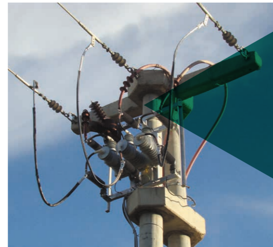
▲ Fuse-switches replacement in Turkey
