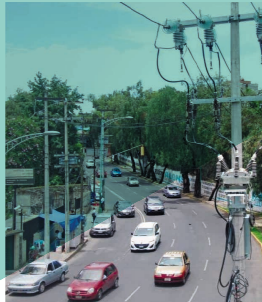
▲ Automatic circuit recloser in the grid automation project in Mexico city
